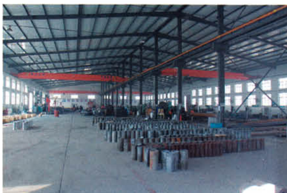
Workshop of pump liner
